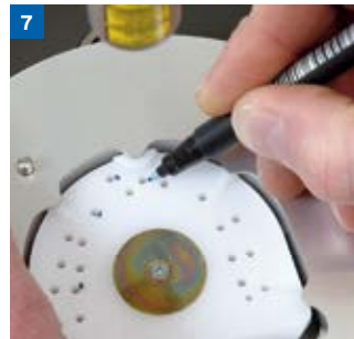
7 Mark out the selected drilling hole on used base plate (multiple usages)
